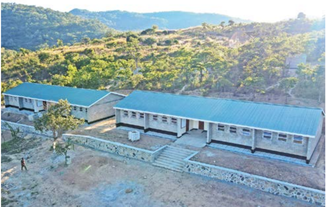
Chiyola Community Day Secondary School under construction
