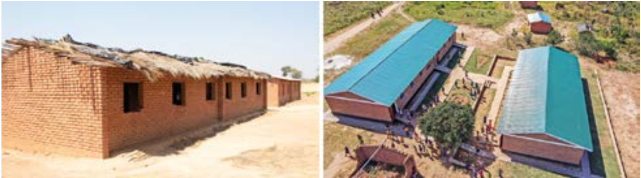
Before and after classroom construction at Balabanthi primary school in Nkhota-kota
