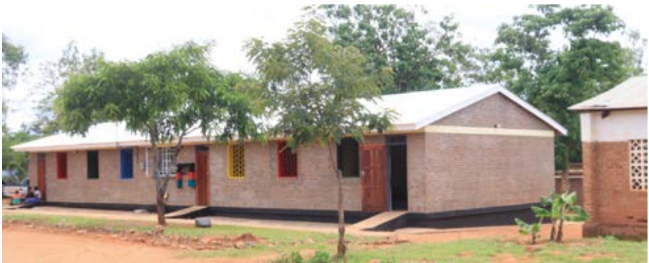
Newly built classrooms at Engucwini Primary School in Mzimba District
